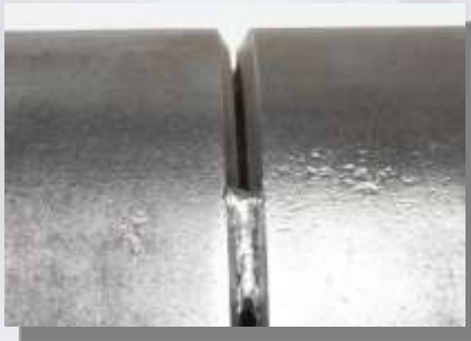
Steel Pipe – Tack Welded
