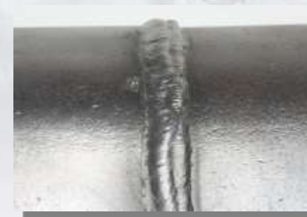
Final weld after several beads are made
